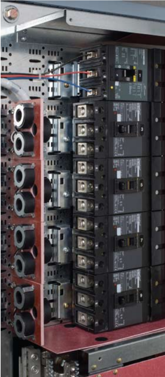
CT mounting configuration for three-phase breakers
