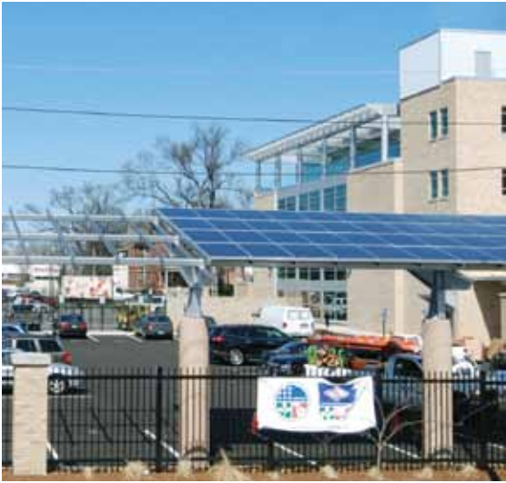
> Solar panels partially installed on-site at state building
