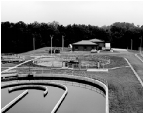
The wastewater treatment facility in McCormick, South Carolina.
